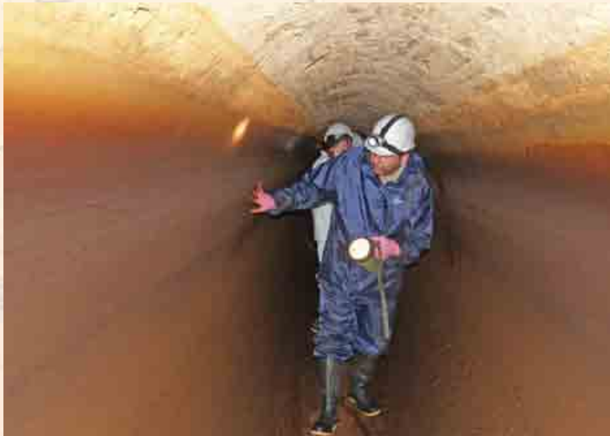
Inspection of the Alviela aqueduct
