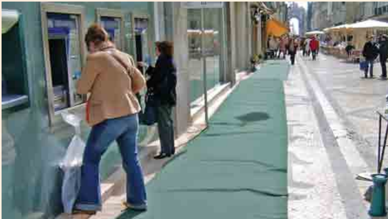
Pavement covering for enhanced pedestrian comfort during works
