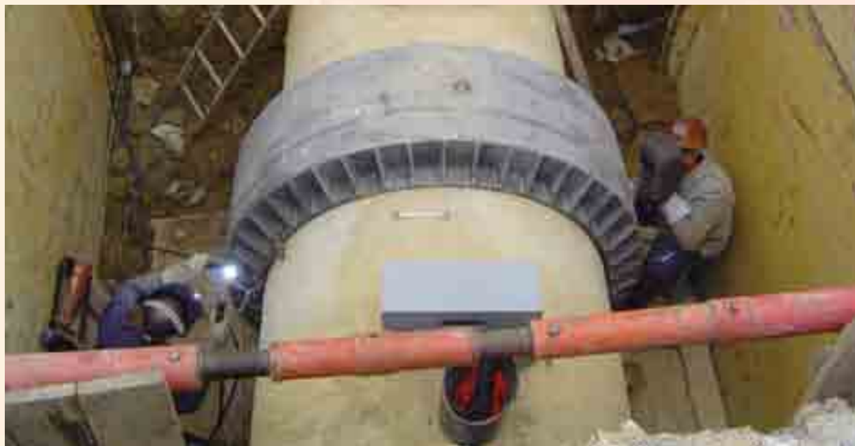
Repair of Ø 1,000 concrete main – placement of ring
